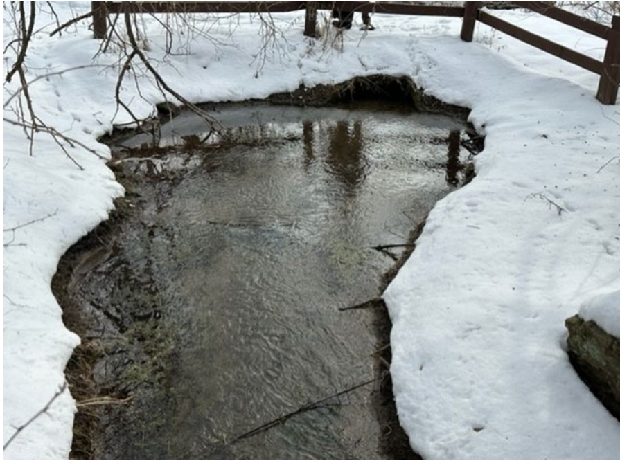
Photograph 2. Upstream view of culvert.
