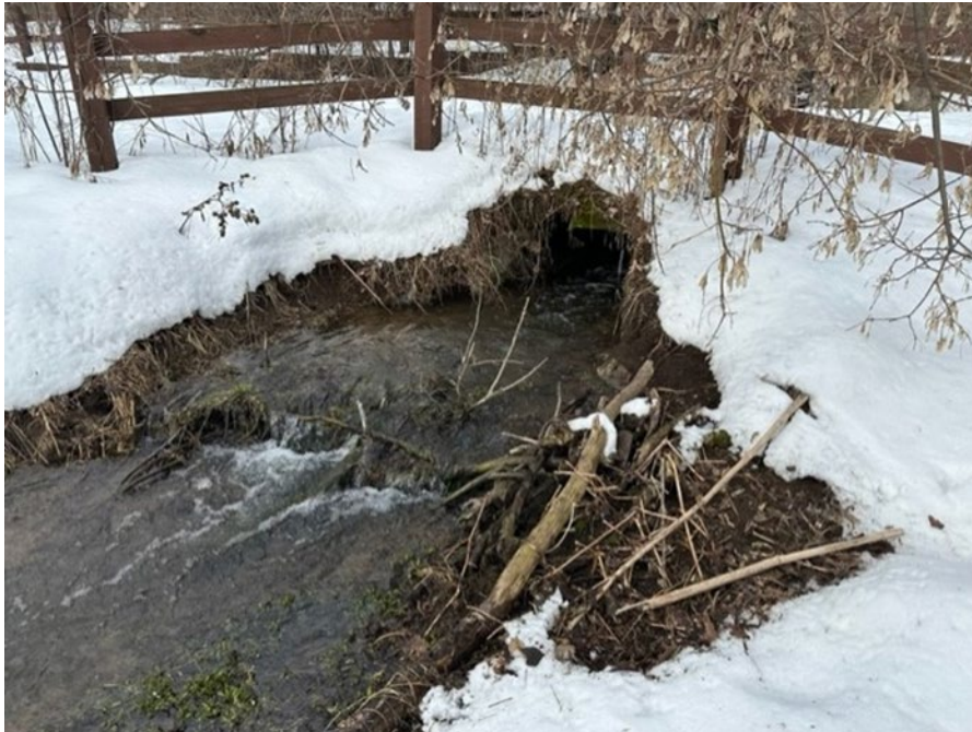
Photograph 1. Downstream view of culvert.
