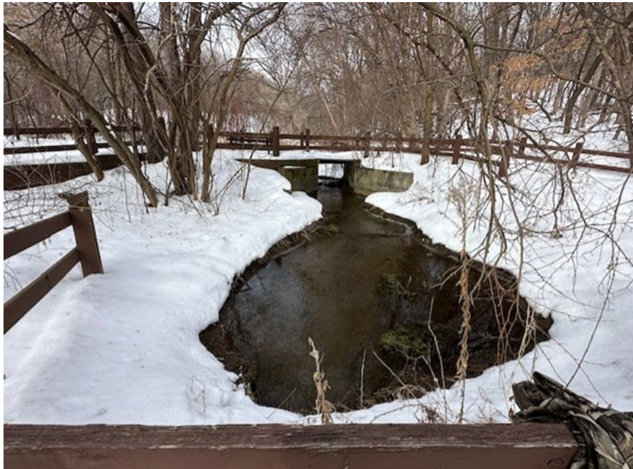
Photograph 3. Control structure looking upstream from culvert.
