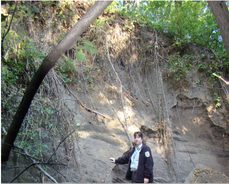
Photograph 5. One example of ravine erosion within the watershed.
