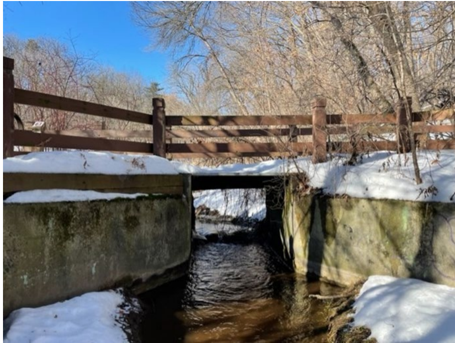
Photograph 4. Control structure close-up looking upstream from culvert.
